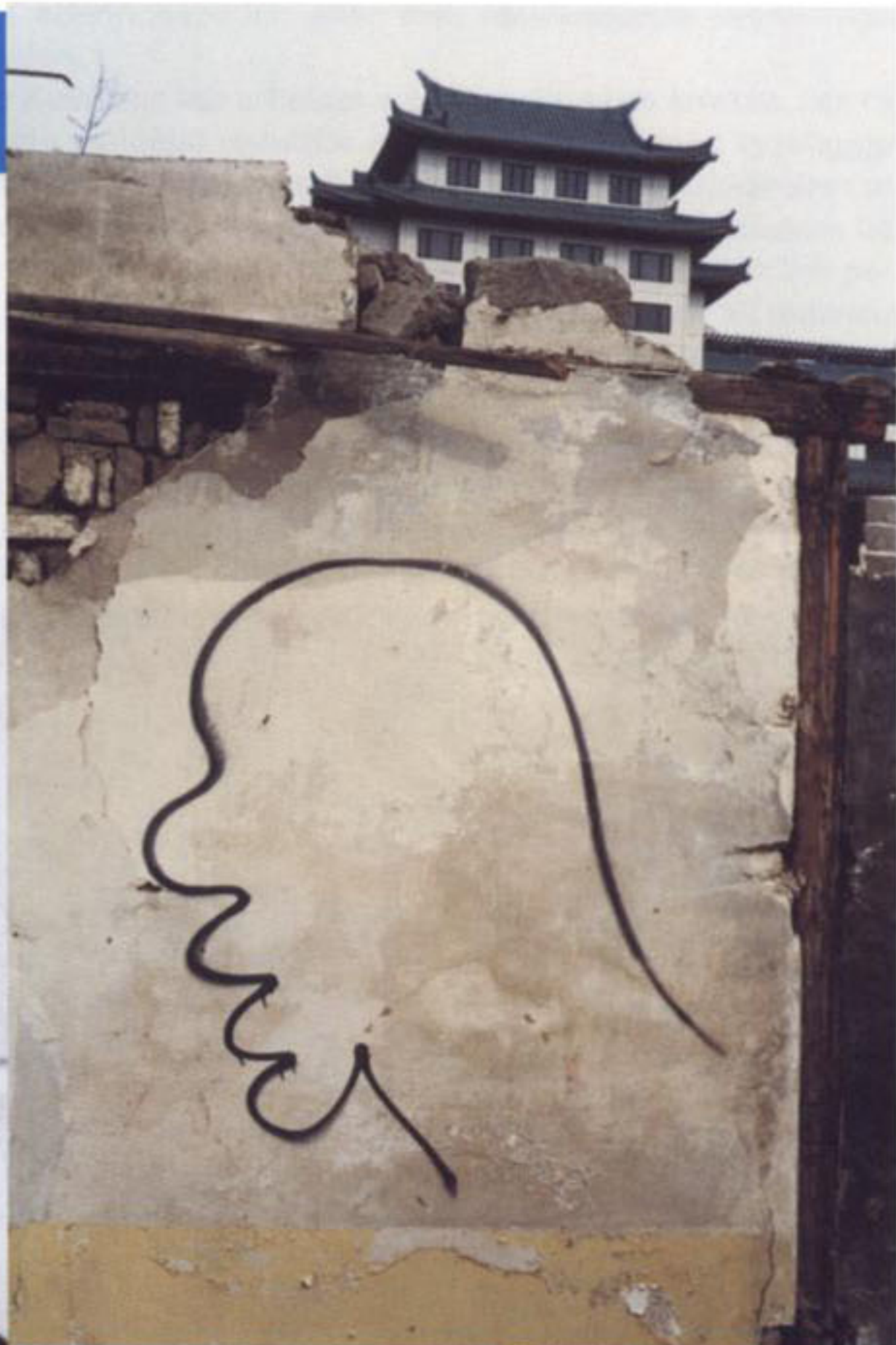
Demolition, World Financial Centre, Beijing, 1998
