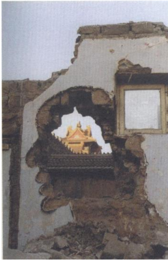
Figure 11. Zhang Oali Demolition, Beijing, 1998
