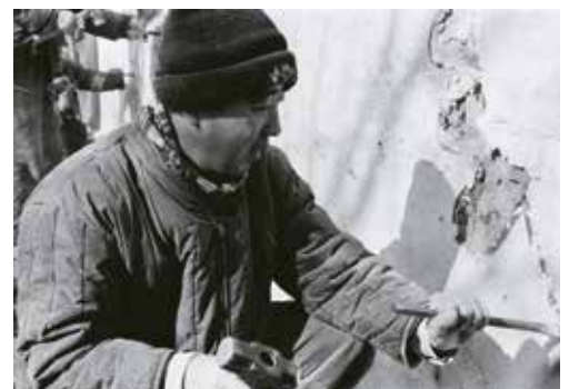
Dialogue and Demolition, Beijing, 1998
