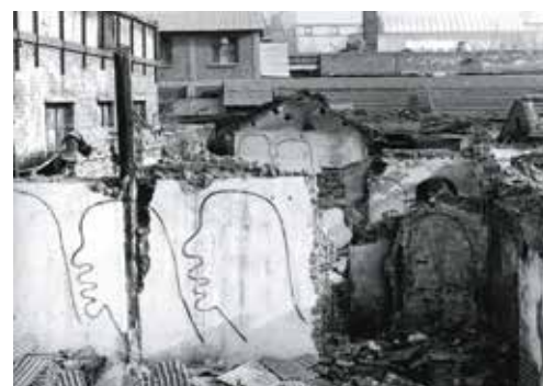
Dialogue and Demolition, Beijing, 1998
